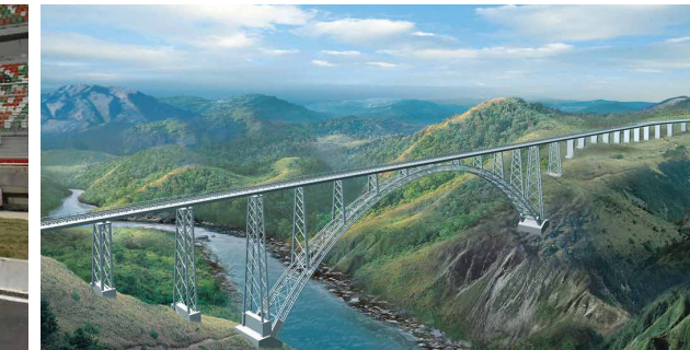
Chenab Bridge - Jammu & Kashmir
