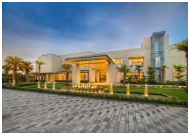
The Aravallis, Sector - 61, Gurugram Ongoing
